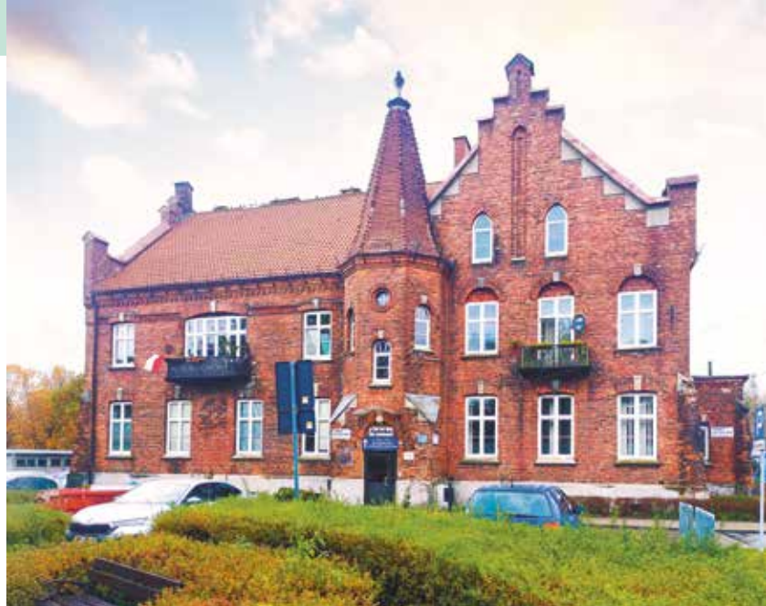
Budynek Szpitala i Ambulatorium | The Hospital and Infirmary Building
