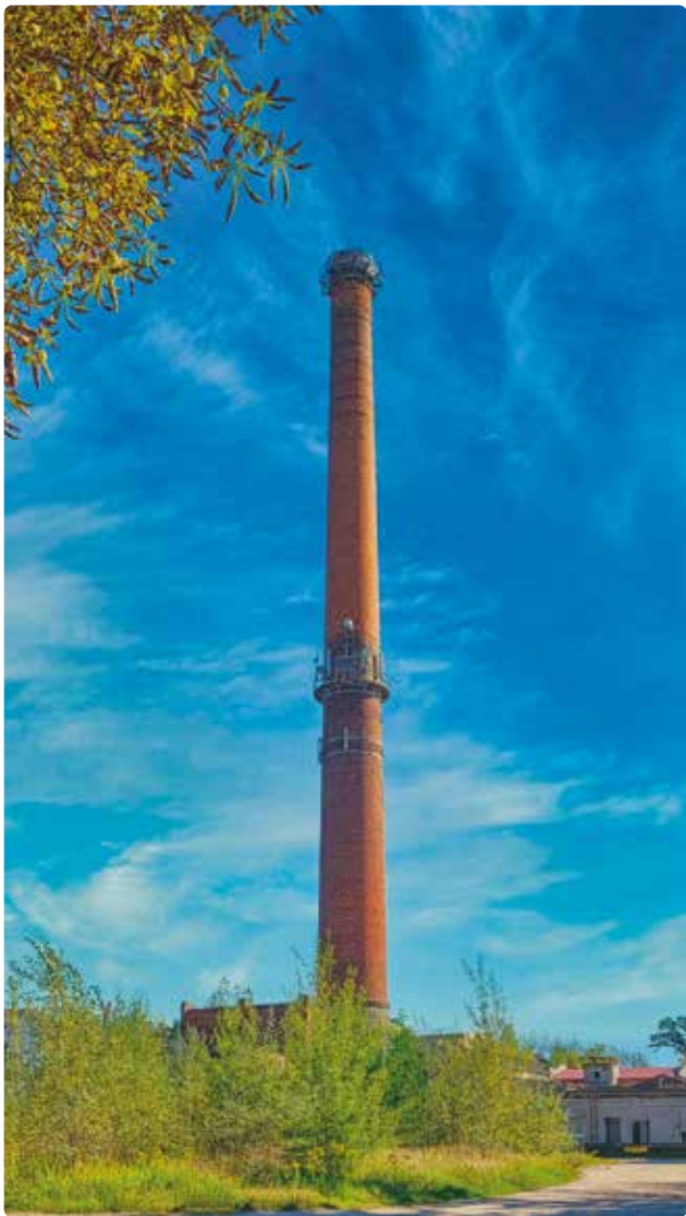
Komin Fabryki Papieru | The Paper Factory chimney
